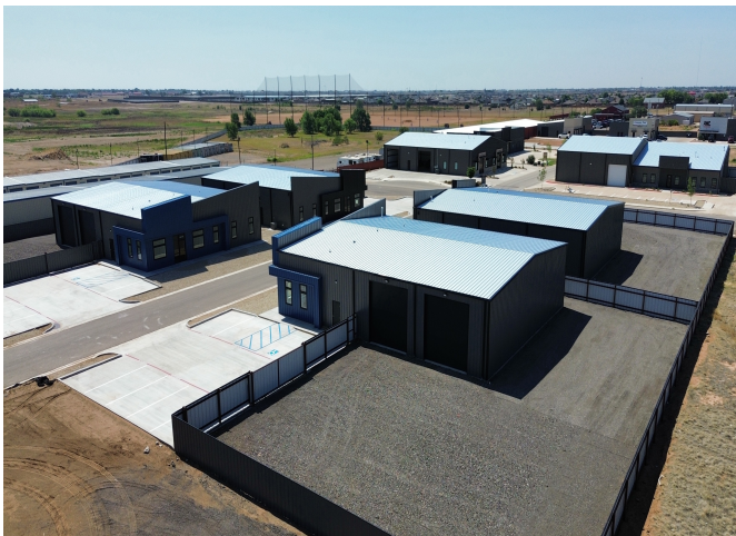
Building yard and fenced storage area
