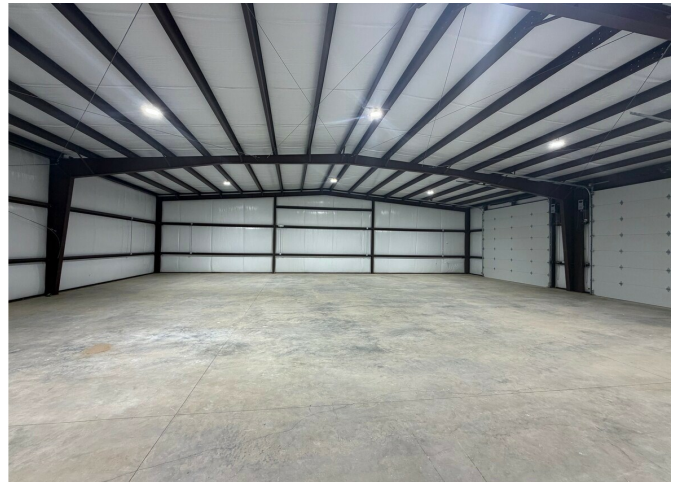
Warehouse — view toward overhead doors
