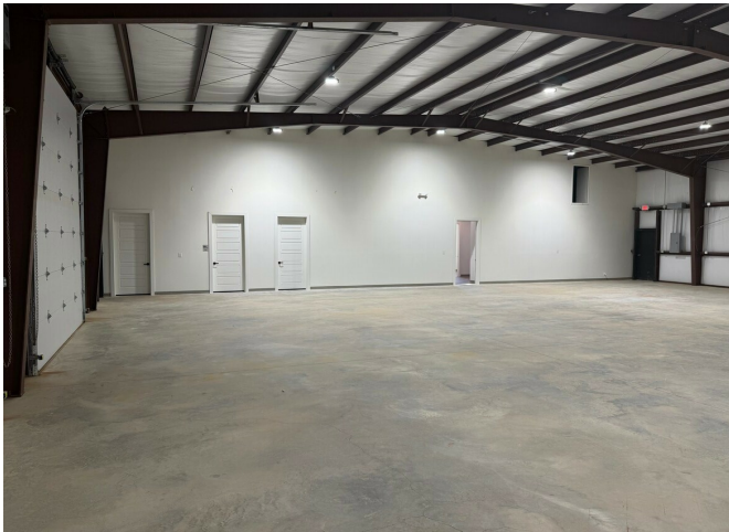
Warehouse interior — open span with LED lighting
