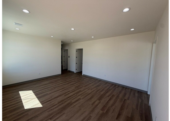
Office suite corridor
