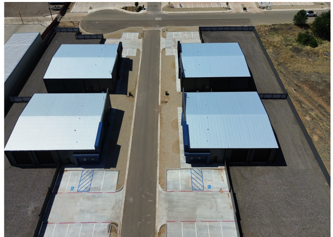
Overhead aerial — all four buildings and parking
