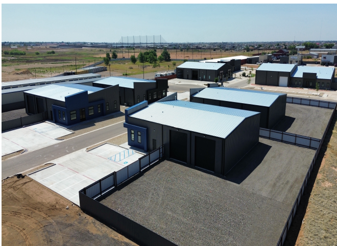
Building yard and fenced storage area
