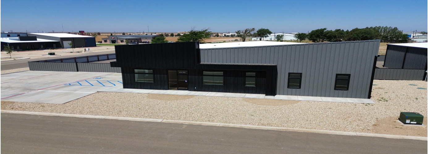
3206 118th Street — street-level front elevation
