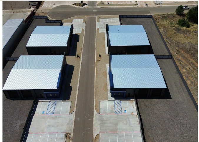
Overhead aerial — all four buildings and parking
