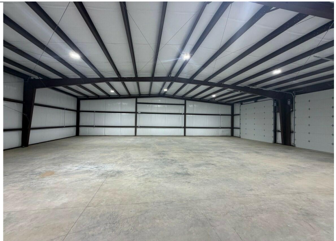
Warehouse — view toward overhead doors
