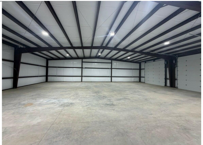
Warehouse — view toward overhead doors
