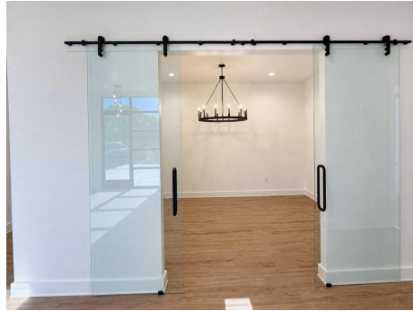
Conference room sliding glass doors
