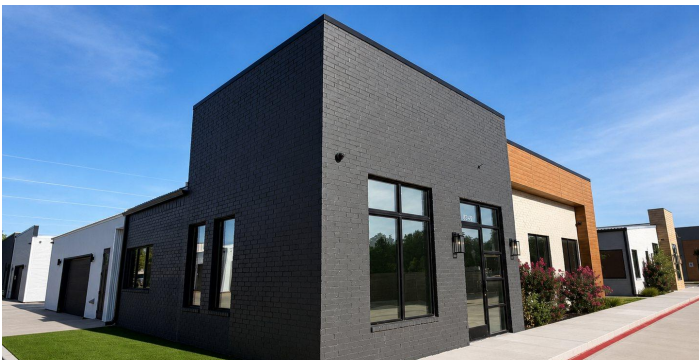
8349 — corner elevation and entry approach
