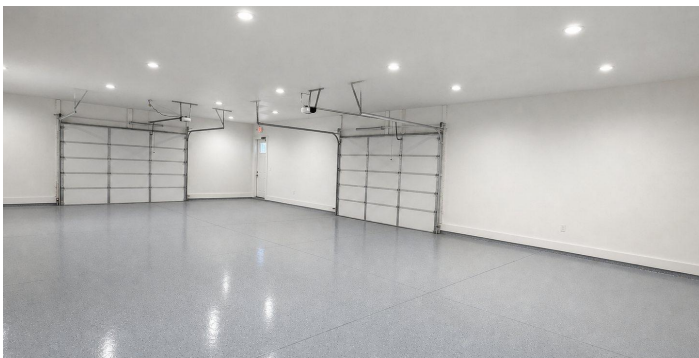
Storage bay — two insulated overhead doors
