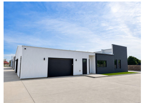
Rear elevation and drive access
