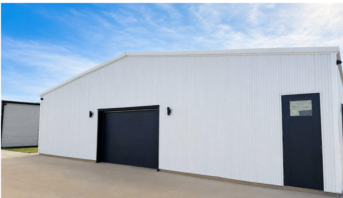
Storage bay — overhead door and service entry
